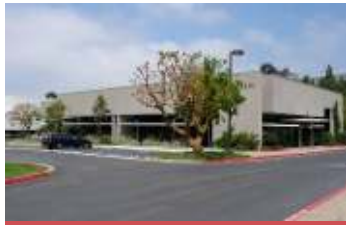
Information Systems Labs 10070 Barnes Canyon Road 30,000 sf
