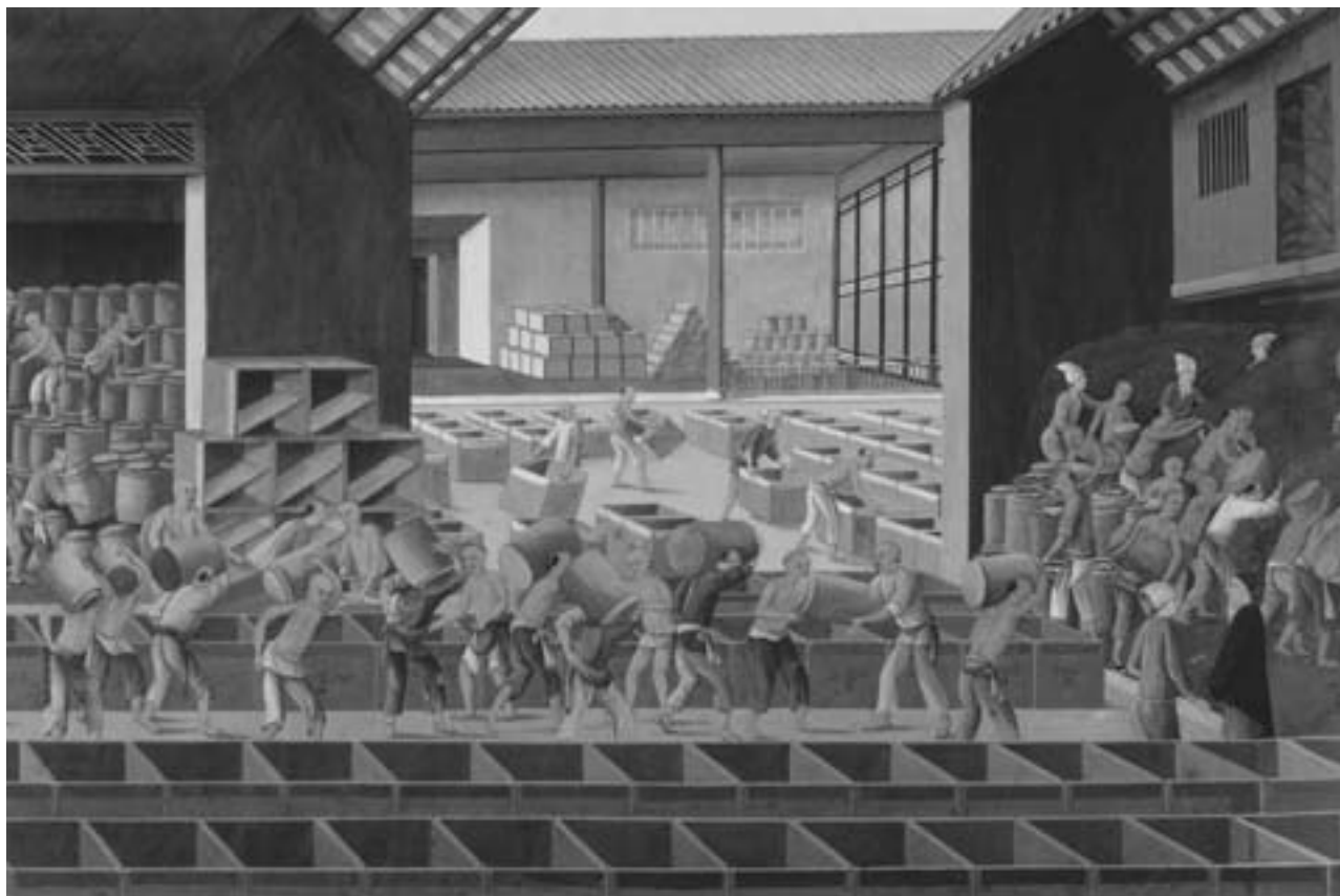
A tea warehouse in Canton (© British Library Board All Rights Reserved 10977)
