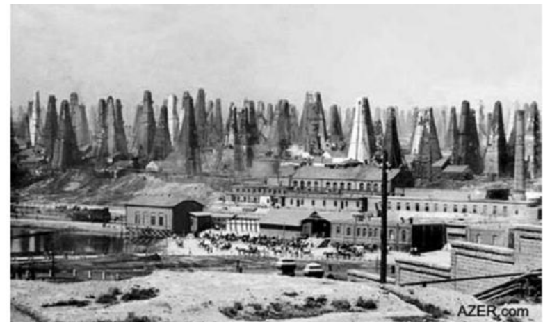
Above: The Nobel Brothers' oil wells in Balakhani, a suburb of Baku. The derricks were so close to each other, making the risk of fire eminent, and the noise level horrendous. Photo: Asbrink Collection.
