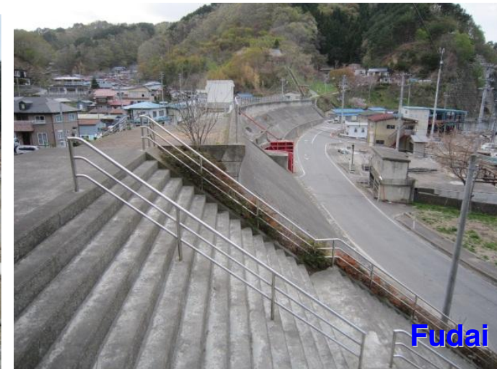
The 15.5m-high seawall was undestroyed in Otabe district, Fudai village, Iwate Pref.
