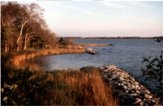
c. Breakwater and sill project after 5 years
