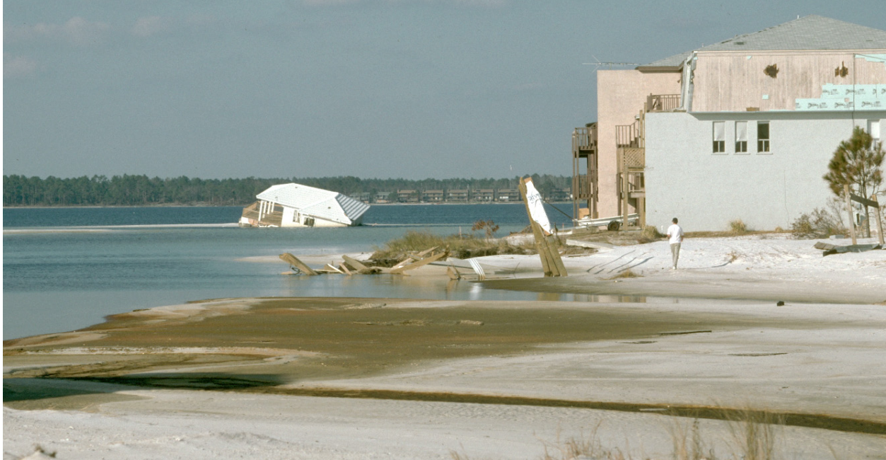
Figure IV-1-13. Navarre Beach, Florida, November 1995. The house in Santa Rosa Sound was lifted off its foundations and moved back hundreds of meters. Many houses here were built on piles, but during Hurricane Opal, some piles were undermined, while at some properties, waves simply lifted buildings up off their supports. The low area in the foreground is a washover channel
