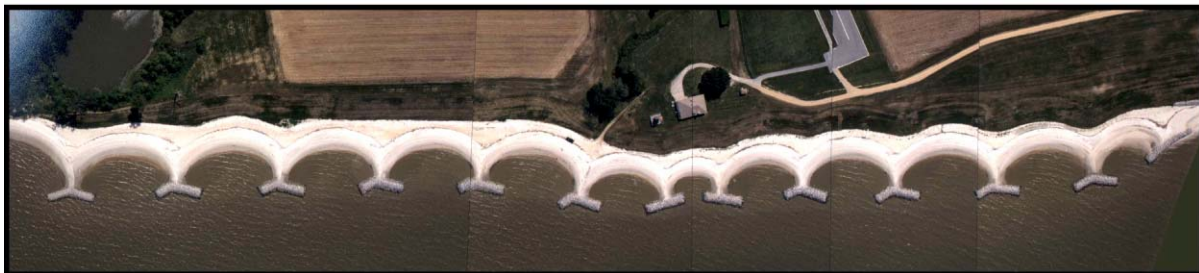
Luter Project One year after construction, May 1999 Approximate photo scale 1 inch=200 ft
