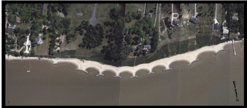
VanDyke Project Two Years After Construction 1999
