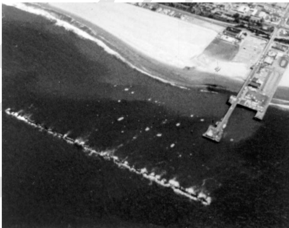
b. Deteriorated breakwater allowing wave transmission
