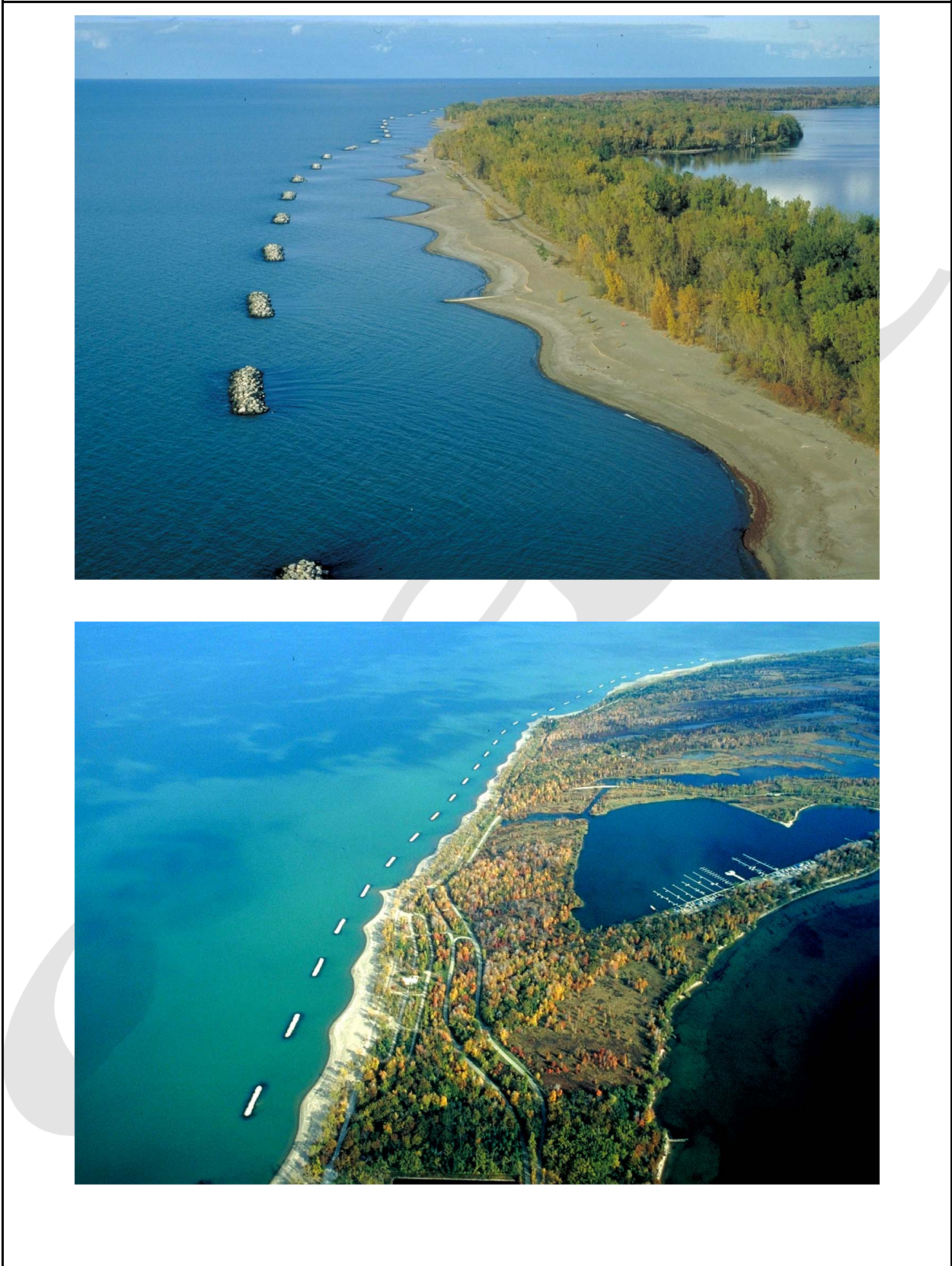
Figure V-3-19. Breakwater construction and salients, Presque Isle, Pennsylvania (from Mohr 1994)
