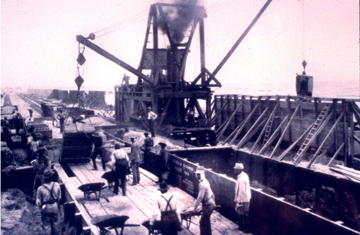
a. Photograph of original construction (from USAED, Galveston)
