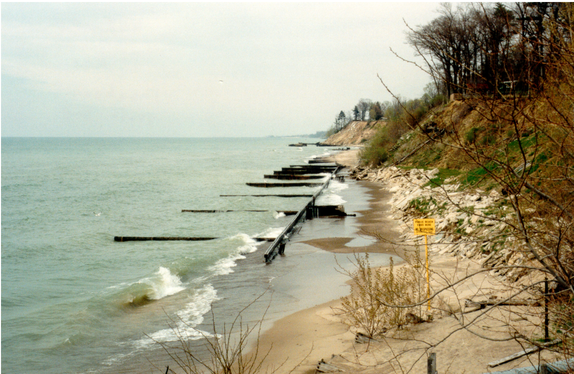
Figure III-5-28. A steel sheet-pile wall and groin field has been ineffective at protecting this section of cohesive shore along the Berrien County shore of Lake Michigan, south of the town of St. Joseph, April 1994
