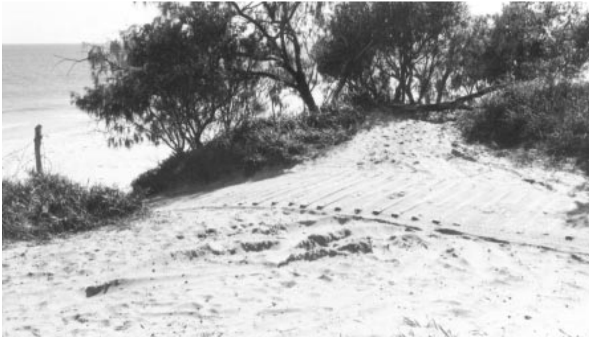
Vehicle access track using a board and chain roadway on the crest and seaward slope of the frontal dune. This track needs to be fenced to prevent further damage to dune vegetation on each side of the board and chain roadway.
