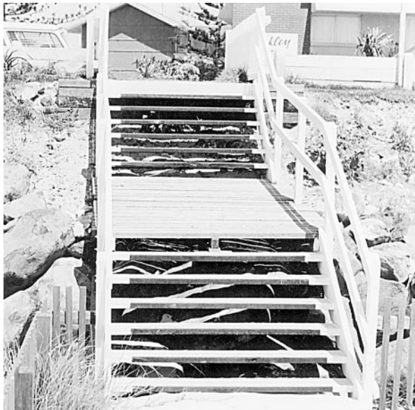
Steps providing access to and from the beach.
