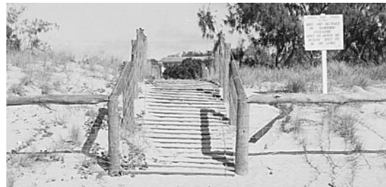
Board and chain walkway and access track to beach.
