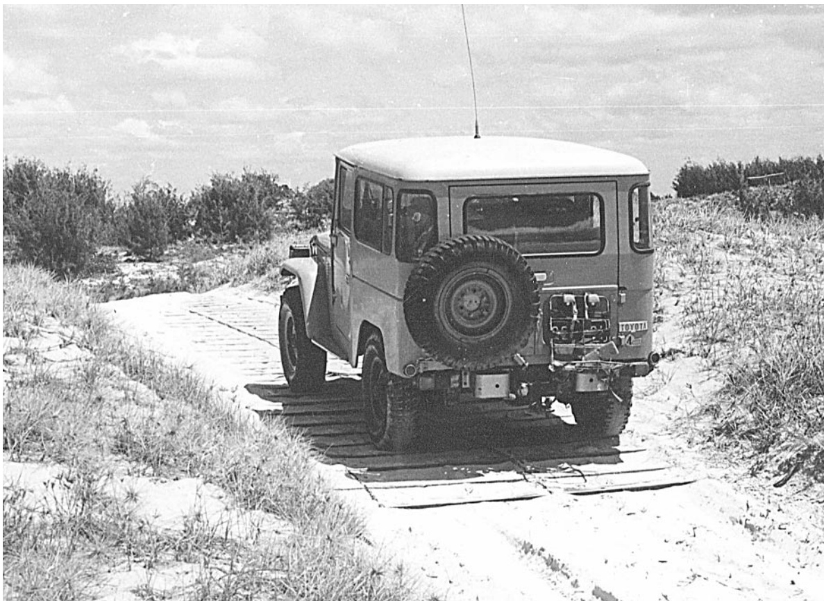
Board and chain roadway in use on a foredune.
