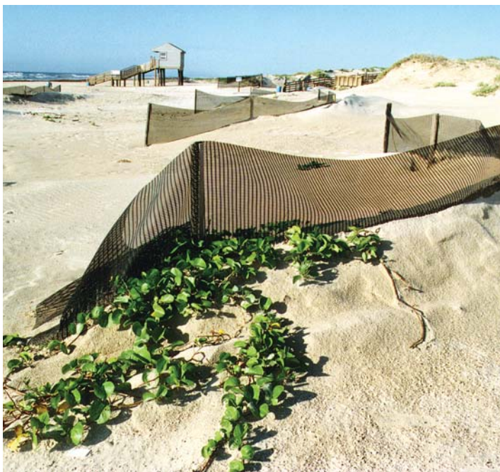
Figure 17. Sand fencing used to trap sand.
