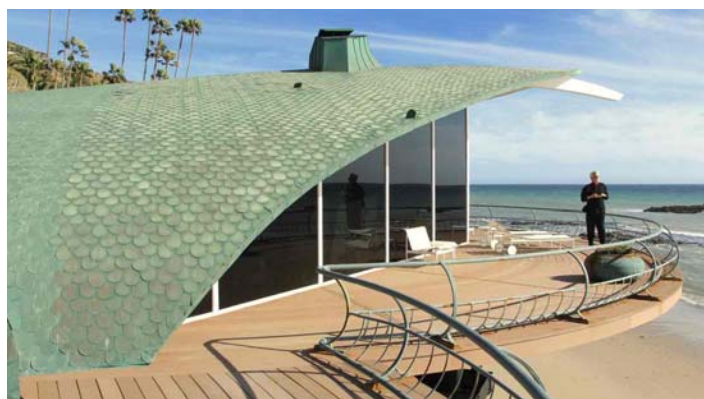
Harry Gesner's Wave House, said to be the inspiration for Sydney Opera House. Photograph: Jordan Riefe
