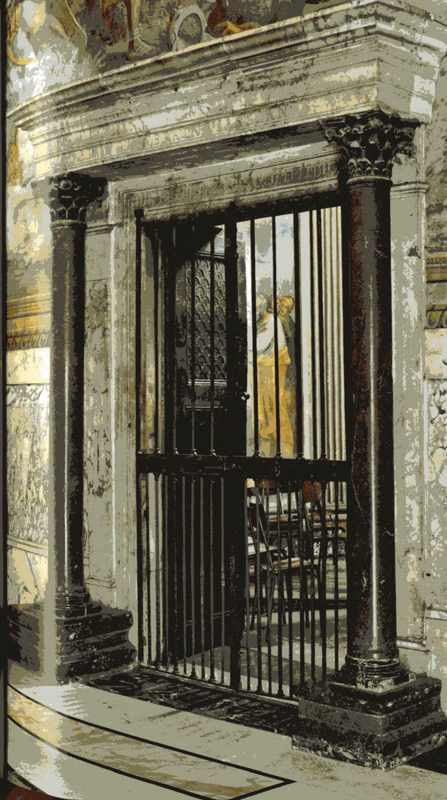
45 The Hilary Chapel (Capella del Battista) with porphyry columns supporting a marble trabeation. The bases and Corinthian capitals are of green porphyry (serpentine).
