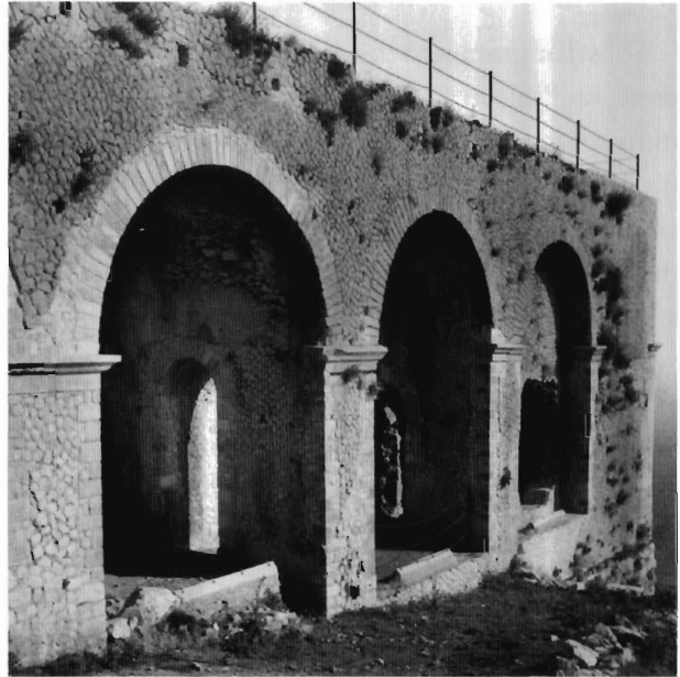
1. Sanctuary of Jupiter Anxur (first half of the first century B.C.). View of concrete vaulted platform overlooking the Tyrrhenian Sea at Terracina. Fototeca Unione c/o American Academy in Rome, neg. #5139.
