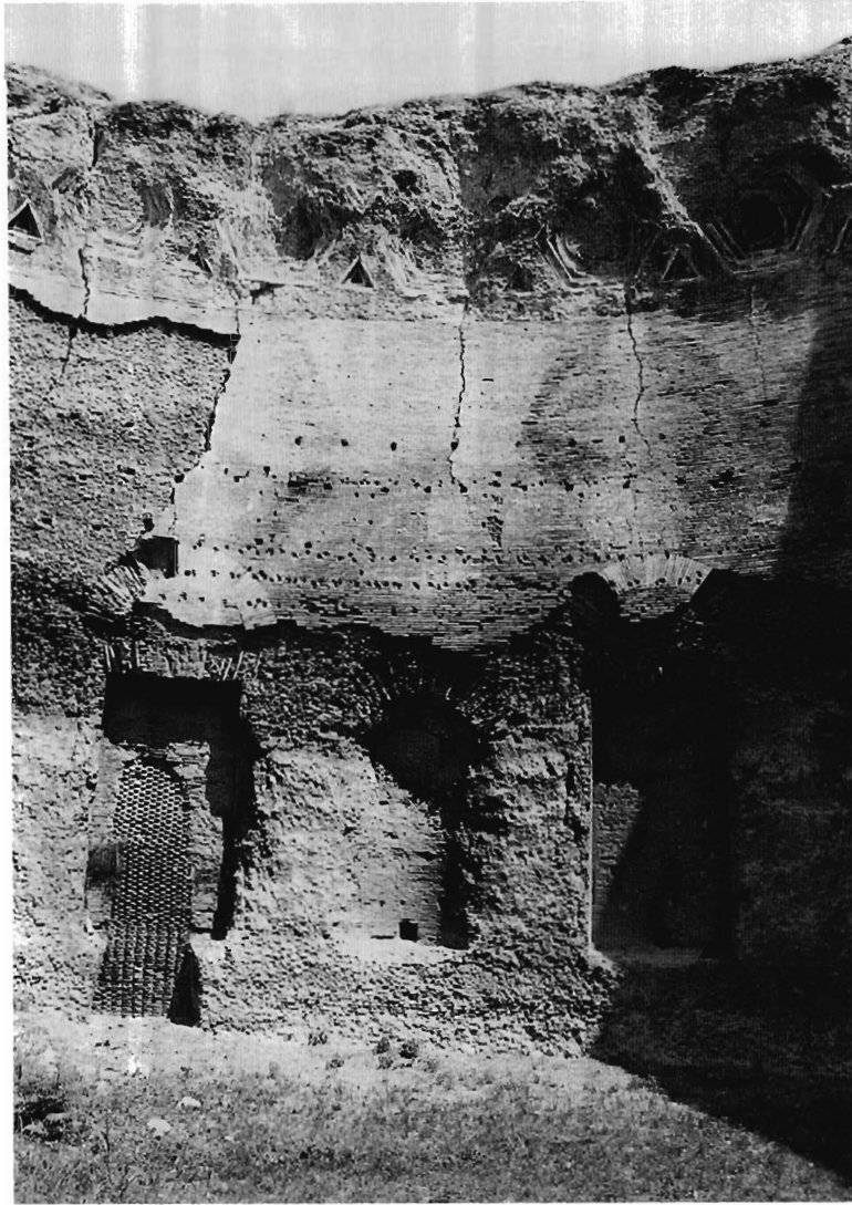
4. Baths of Trajan (A.D. 104–109). Detail of the exedra at section D showing cracks in wall supporting semidome (29.5-m span).
