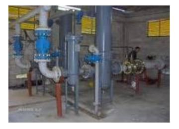
If the maximum pressure allowed is 25 bar, the system must be placed against the wall of fence enclosing the area of the property, and if between 5 and 25 bar must be located as far away as possible from buildings or warehouses.
