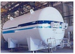
The cryogenic fuel is a fuel that requires to be stored at extremely low temperature to enable it to maintain the liquid state. They are, in fact, generally constituted by the liquefaction of gases such as, for example, liquid oxygen. It is mistakenly called "cryogenic fuel", but it is more correct to identify it as oxidizing and not as a fuel.
