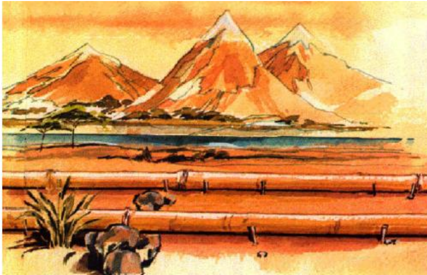
Fig 1. First pipeline made by bamboo in China about 1000 B.C. [1]
