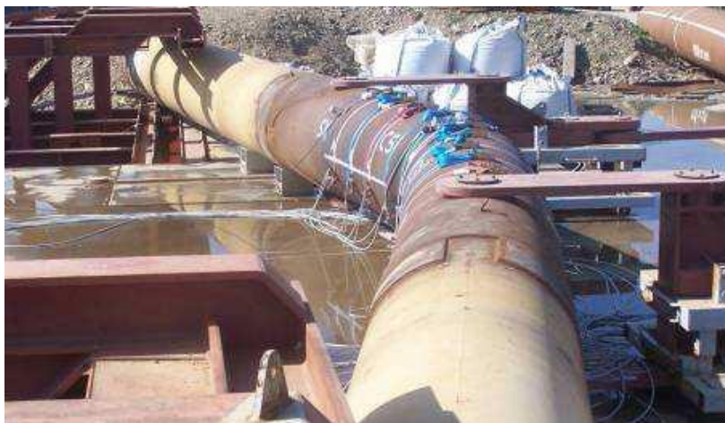
Fig.7b. View of a Pipe Section after the Bending Test
