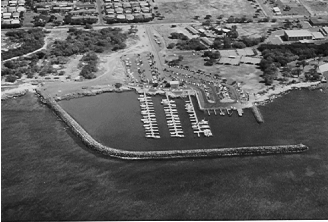
Figure V-5-31. Harbor with shore-connected breakwater, Waianae Small Boat Harbor, Oahu, Hawaii (June 198)
