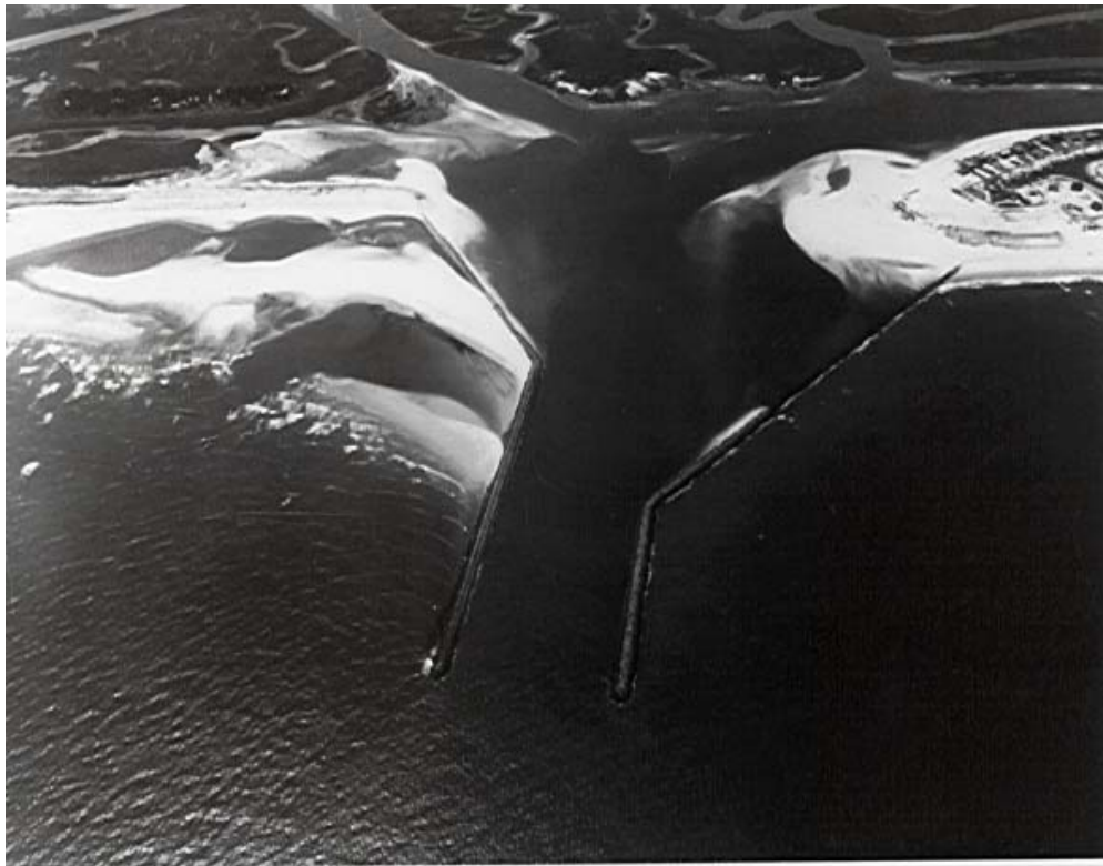
Figure V-5-36. Dual jetty configuration at a tidal inlet, Murrells Inlet, South Carolina (March 1982)
