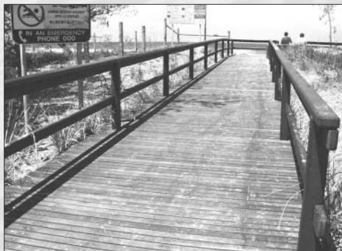
Timber boardwalk providing pedestrian and wheelchair access to a beach viewing platform.
