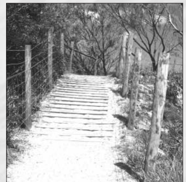
Board and chain is the preferred pedestrian access track surface over the fore-dune crest and down onto the beach.
