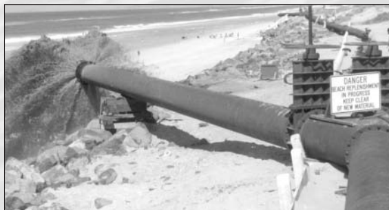
The early stages of re-establishing a beach and dune system with sand dredged from a nearby estuary.
