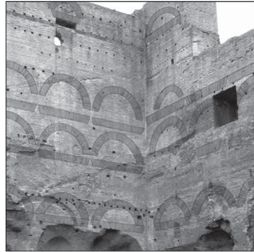
Fig. 3: Domitianic Vestibule, Palatine. Series of relieving arches in walls.
