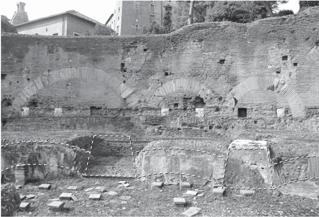
Fig. 6: Trajanic Latrine at the Forum of Caesar. Photo of springer blocks directing loads to underlying vaulting ribs.
