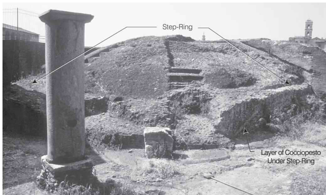
Fig. 11: Trajan's Markets. Step-ring on extrados of the semidome at the north end of hemicycle.
