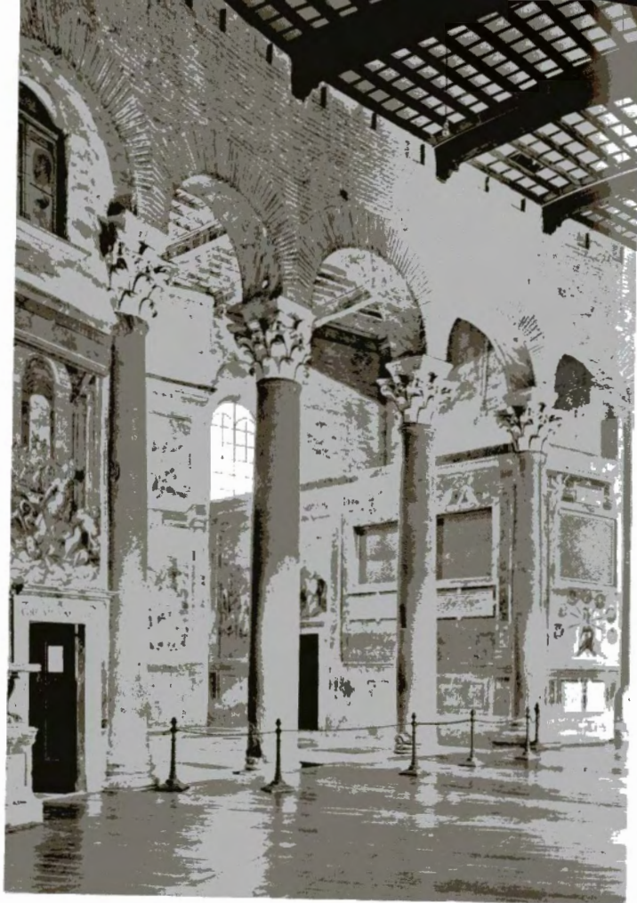
106 Santo Stefano Rotondo: four spolia columns with granite shafts and Corinthian full-leaf capitals (late third century) separating the ambulatory from what was originally the north-eastern narthex .
