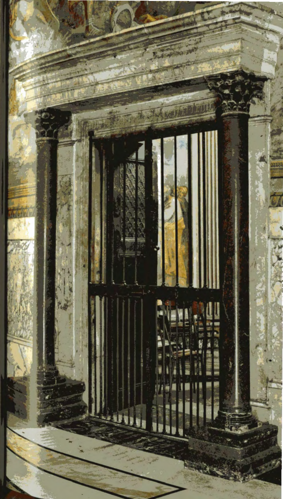
45 The Hilary Chapel ( Capella del Battista ) with porphyry columns supporting a marble trabeation. The bases and Corinthian capitals are of green porphyry (serpentine).
