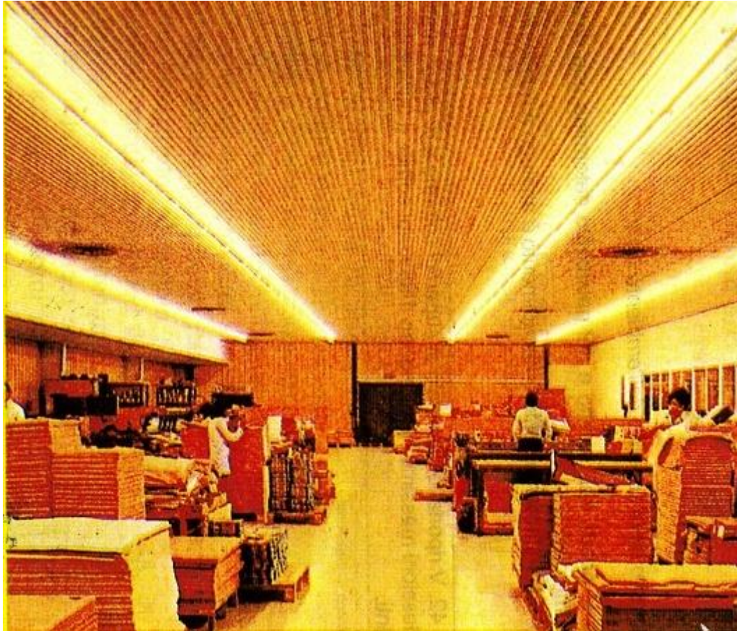
Lighting fluorescent tubes in a textile company
