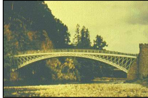
Telford's Mythe Bridge 1823-26 (52m)
