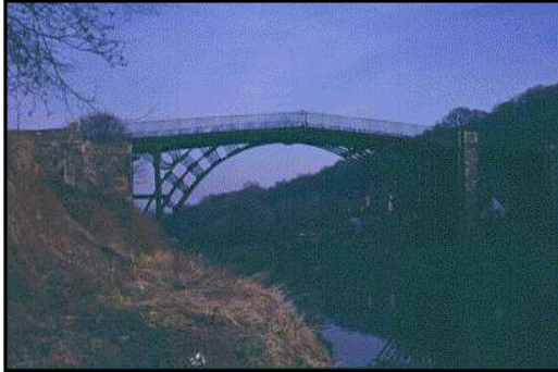
Coalbrookdale bridge sul Severn 1779 (33m)
