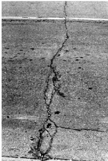
FIG. X1.23 Medium-Severity Joint Reflection Cracking
