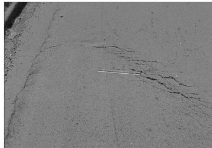
FIG. X1.48 Medium-Severity Slippage Cracking
