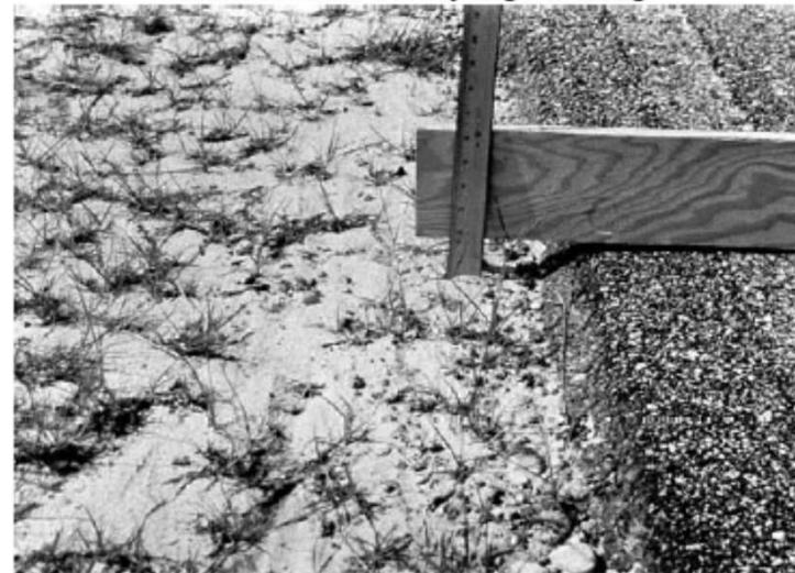
FIG. X1.25 Low-Severity Lane/Shoulder Drop-Off
