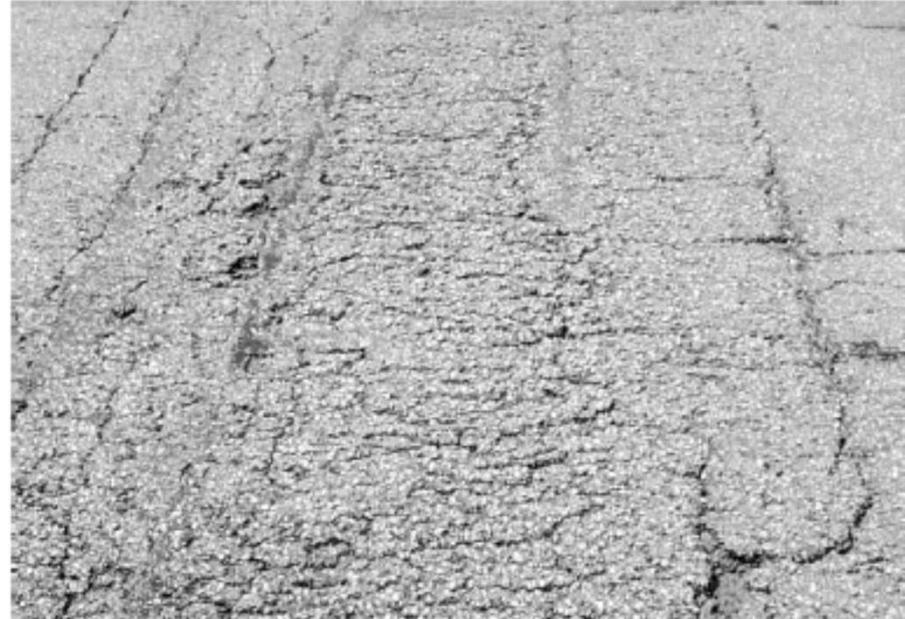
FIG. X1.52 Medium-Severity Weathering and Raveling
