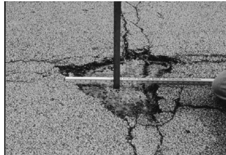
FIG. X1.36 Medium-Severity Pothole
