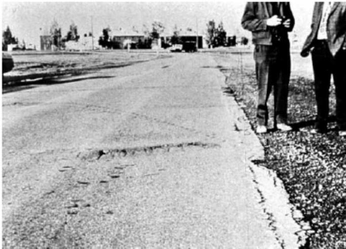
FIG. X1.11 Medium-Severity Bumps and Sags
