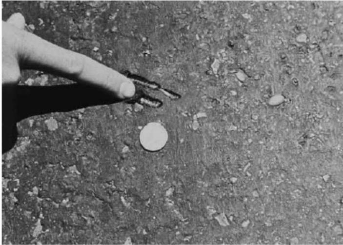
FIG. X1.5 Medium-Severity Bleeding
