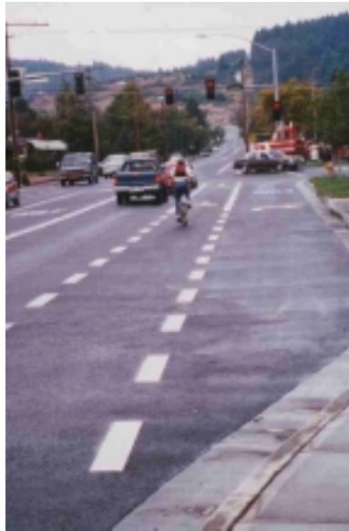
ILLUSTRATION 11-4. Bicycle lane treatment at a signalized intersection.
