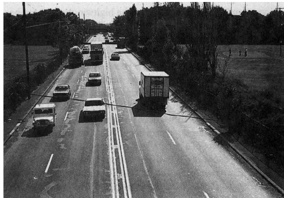
ILLUSTRATION 12-6. Inadequate shoulder width and other obstructions along multilane highway.
