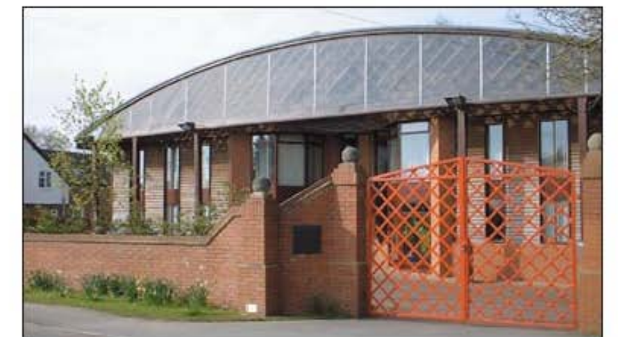
Architectural merit of the single span timber roof – Lattice House
