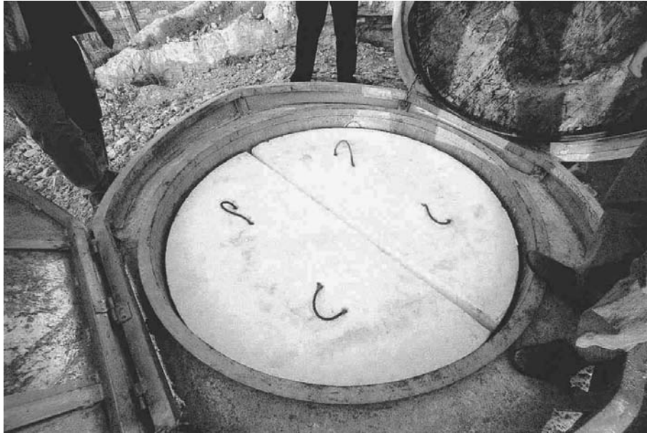
Fig. 7.41 Thermal cover of a seismic vault in two pieces made of thick styrofoam. The gaps between the cover and the vault walls and between both pieces must be tightly sealed.
