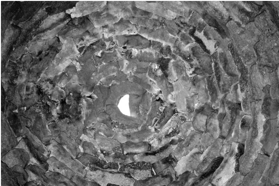
4.11. Nuraghe “Is Paras,” near Ìsili, Sardinia, detail of corbeled dome. (Photo author)
