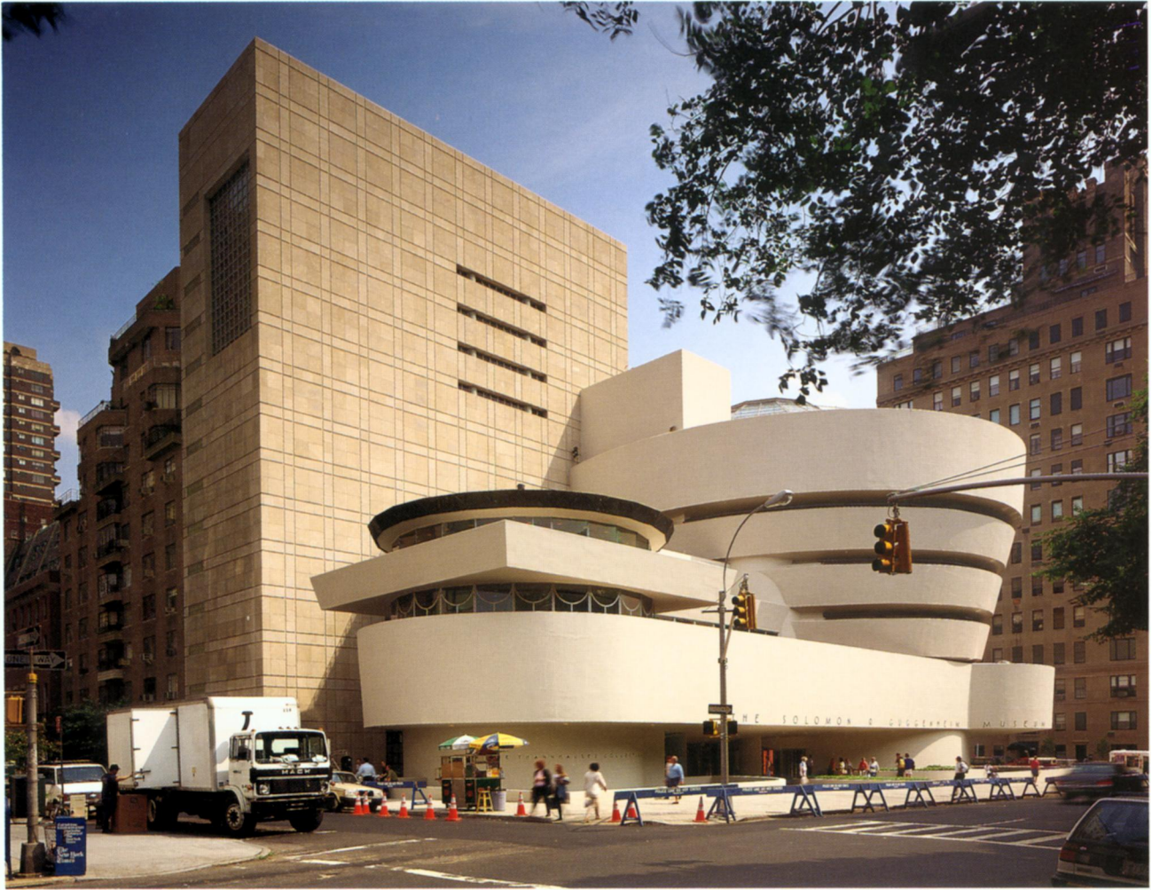
Fig. 26. Frank Lloyd Wright, The Solomon R. Guggenheim Museum. Elevation from Fifth Avenue with additions and renovations by Gwathmey Siegel & Associates. (© Jeff Goldberg/Esto. All rights reserved.)
