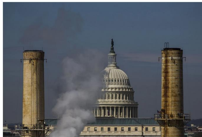
The dome of the U.S. Capitol is seen behind the smoke stacks of the Capitol Power Plant, the only coal-burning power plant in Washington, D.C.
