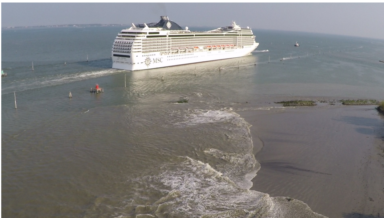
Fig 5. Aerial view of a cruise ship transit in the MMC. The depression wake exposes the collapsed materials of the original rip-rap revetment of the embankment at the southern end of the Cassa di Colmata B (CC-B). Image source: author's picture.
