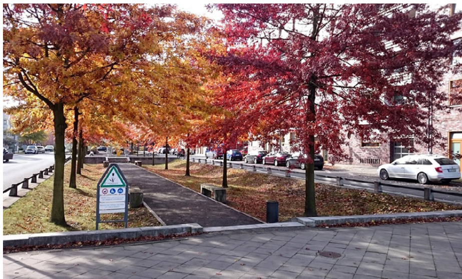
Figure 11. Trough infiltration system in the Rummelsburg district of Berlin. Rainwater is temporarily stored in a permanently green trough, which is then emptied by means of infiltration and evaporation.
