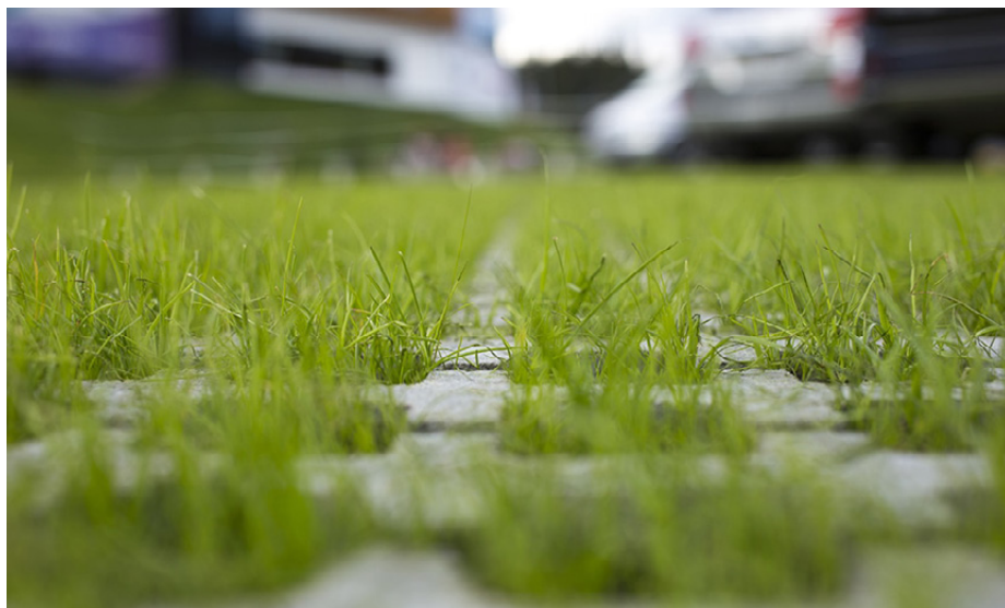
Figure 19. Permeable paving is a valuable and ecological alternative to traditional asphalt pavements.
