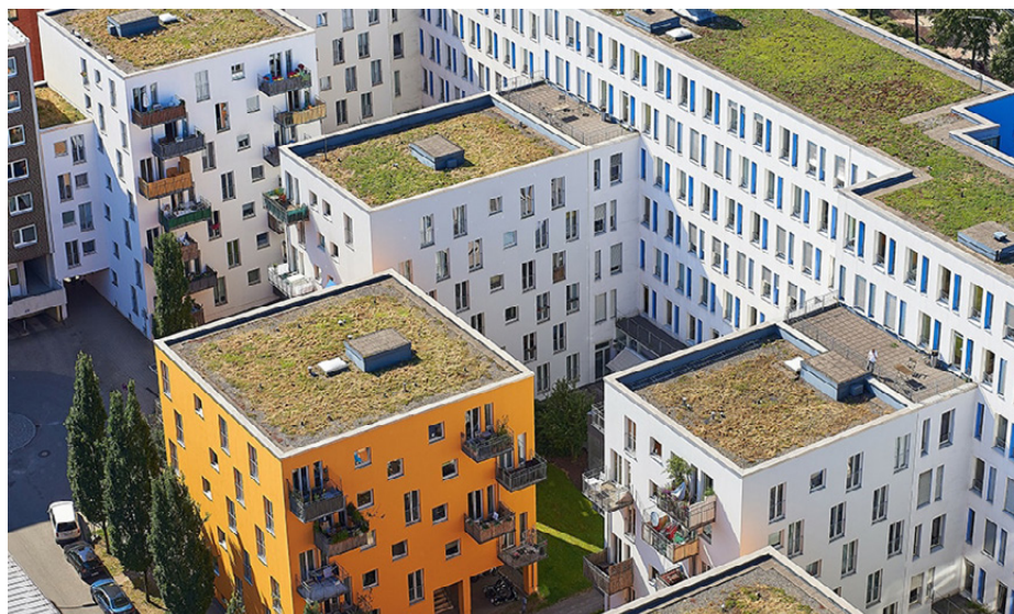
Figure 21. Green roofs in Hamburg.
