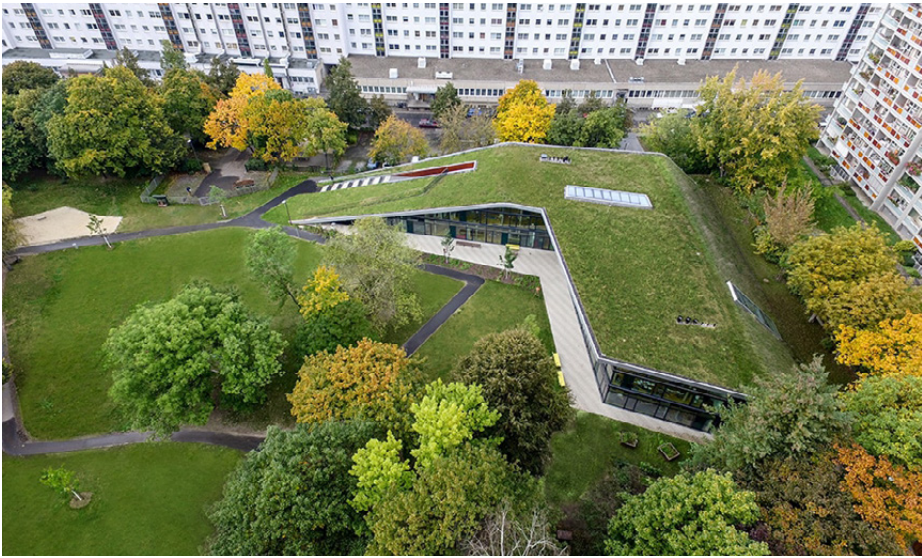
Figure 20. The intensive green roof of the kindergarten building in a Dresden residential area seamlessly connected to the lawns of the surrounding park.
