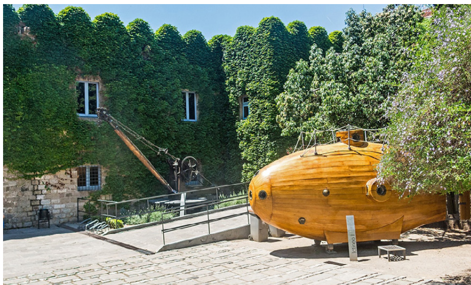
Figure 16. Green walls in the Maritime Museum in Barcelona.
