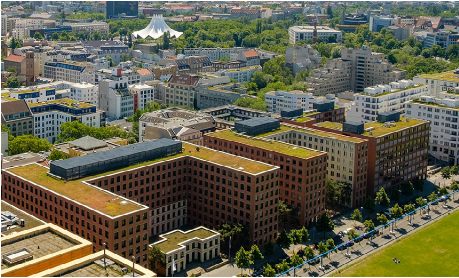
Figure 6. Green roofs in Berlin reduce heat island effect and retain rainwater.
