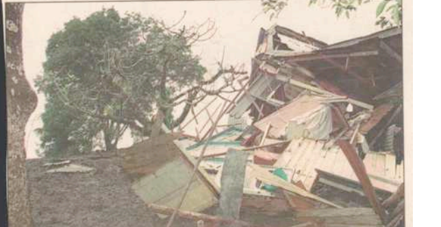
BELOW: A HOUSE is left in ruins in the aftermath of the eruption of a mud volcano in Piparo early yesterday morning. This house was pushed over by the wall of mud on the left. RIGHT: MEMBERS of a Piparo family salvage what is left of their belongings from this second house which was pushed over and partially covered by mud following the early morning eruption. Photo: STEPHEN AJZZ
