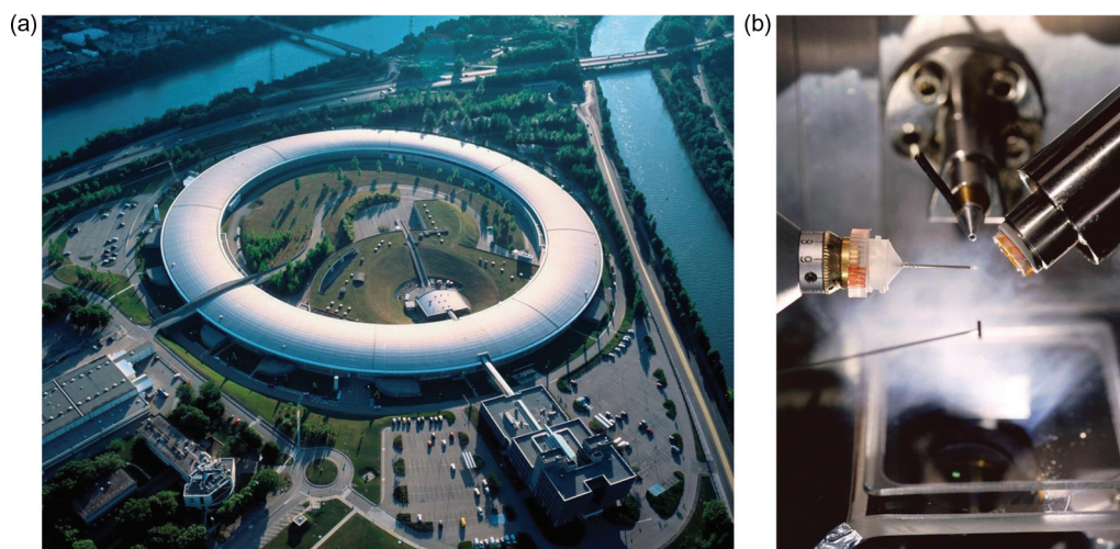
FIGURE 22.8 (a) Aerial view of the ESRF, located between the rivers Isère and Drac in Grenoble, France. Electrons circle around in a large ring inside the circular building, and when they pass bending magnets or assemblies of magnets called undulators they emit powerful X-rays. (b) Crystal being exposed, viewed from the position of the detector. X-rays emanating from the narrow steel tube in the back hit a frozen crystal in the cryo-loop in the center of the picture. The direct beam is stopped by a beam-stop, the small piece of metal just below the center of the picture. On the left is the goniometer, which is used to rotate the crystal, and from the nozzle on the right cold (100 k) nitrogen gas is blown over the crystal. Pictures courtesy of ESRF/Morel.
