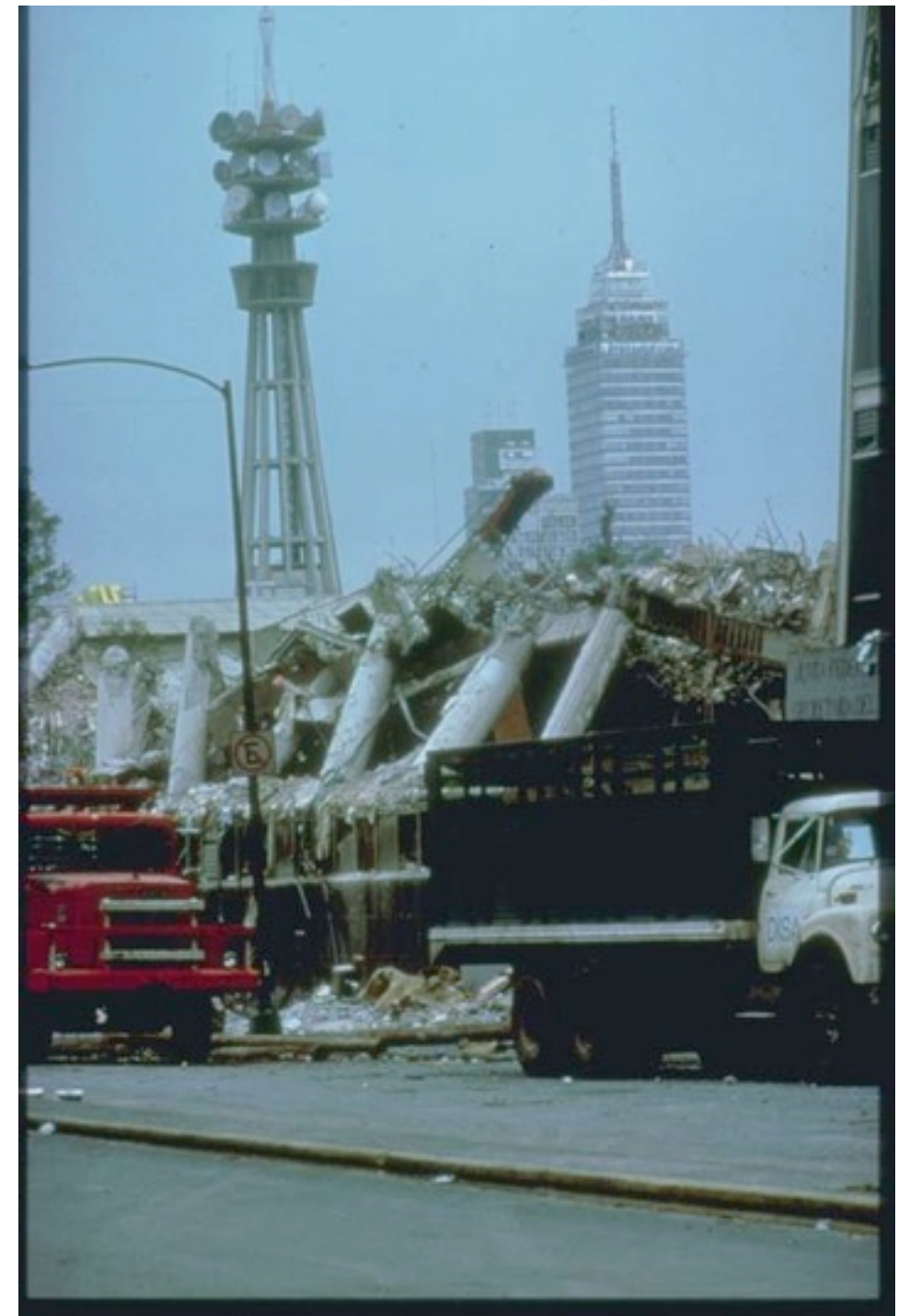
Totally destroyed office building in the foreground, while the 44-floor Torre Latinoamericana office building, in the background on the right, stands
