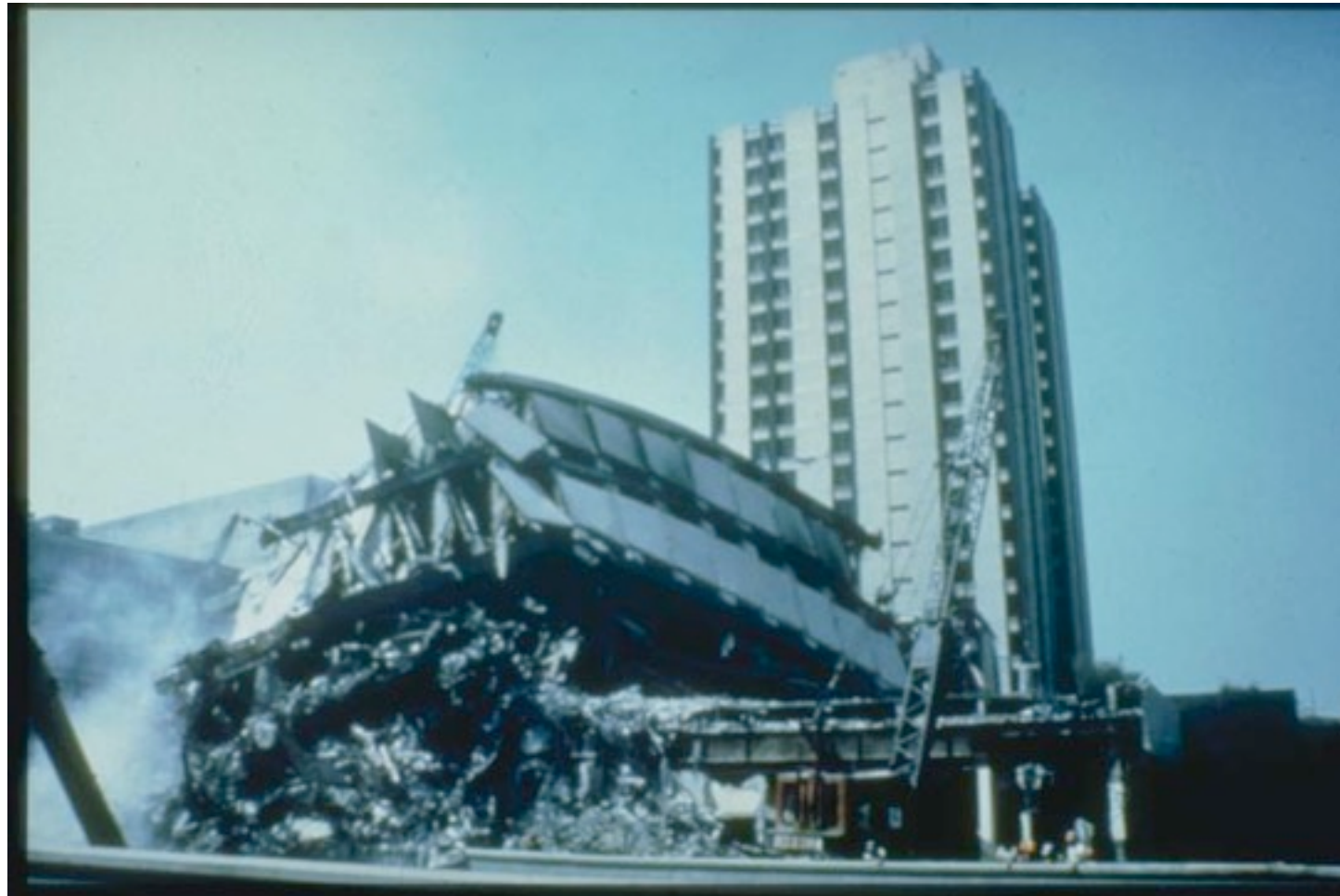
Wreckage of a twenty-one-story building in Conjunto Pino Suarez Complex
