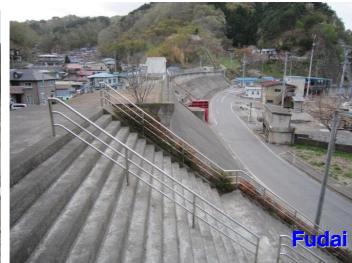
The 15.5m-high seawall was undestroyed in Otobe district, Fudai village, Iwate Pref.
