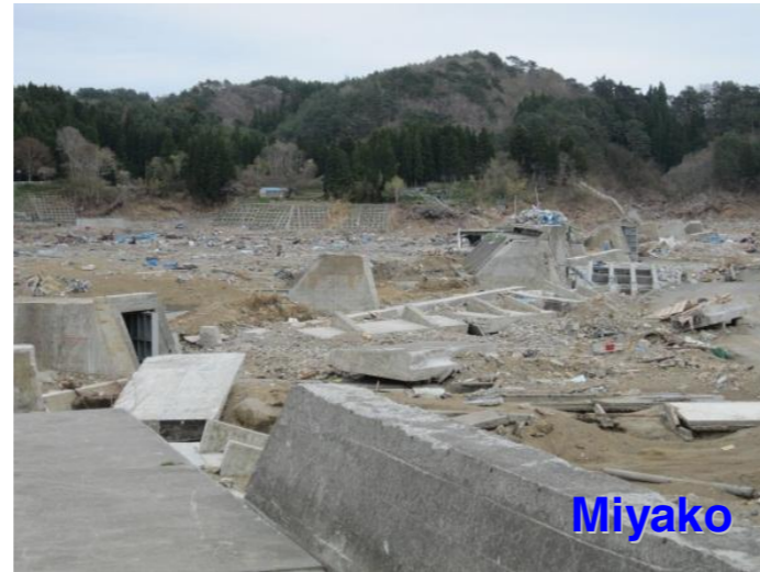
The 10m-high seawall was destroyed in Taro district, Miyako city, Iwate Pref.
