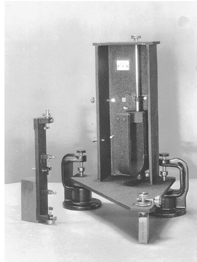
One clever variation on this basic seismometer design was developed in southern California by Harry O. Wood and J.A. Anderson, who invented the "torsion seismometer" in 1922. The motion generated when this instrument was shaken by an earthquake came not from a suspended pendulum, but from the torsional (rotational) motion of a small inertial mass affixed to a thin wire under high tension.
