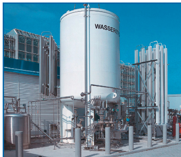
Figure 10 Medium-scale industrial liquefier. Courtesy of Linde Gas.
