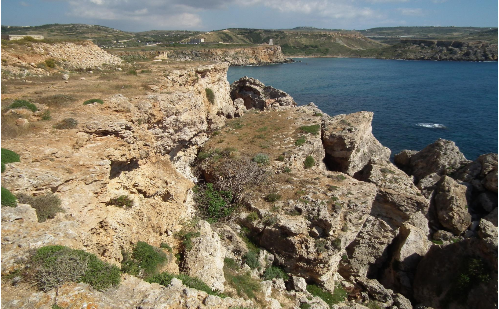
Photo: Lowered blocks detached and moved by rock spreading phenomena
