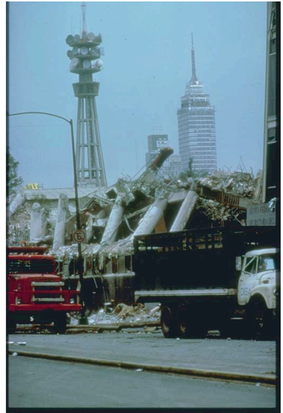
Totally destroyed office building in the foreground, while the 44-floor Torre Latinoamericana office building, in the background on the right, stands
