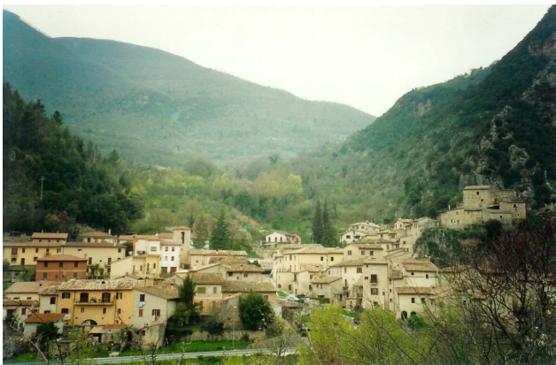
Fig. 5. Piedipaterno village, built on the Lagarelle creek alluvial fan.
