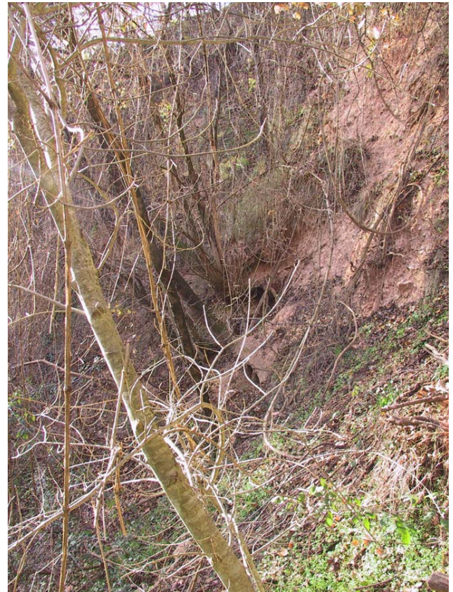
Fig. 8. Banks instabilities along the channel (tract 2).
