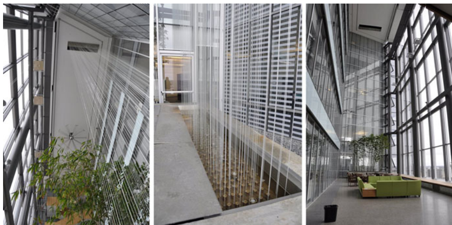
Fig. 7.10 Left : tall water curtain wall, Middle : water ribbons, Right : winter garden atrium space, © photos by Terri Boake
