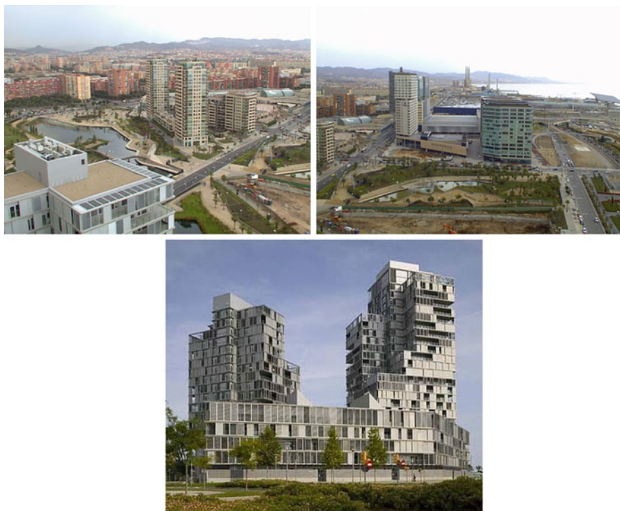
Fig. 10.6 High-rise buildings in a marine environment
