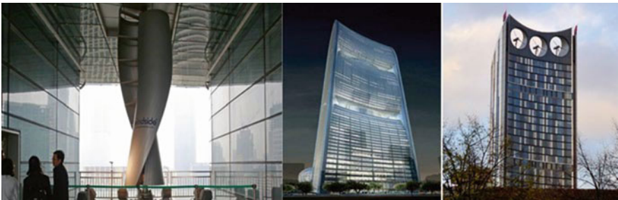
Fig. 6.4 From left Integrated wind turbine in Pearl River Tower (courtesy SOM), Pearl River Tower in China (courtesy SOM), Strata SE1 project in London
