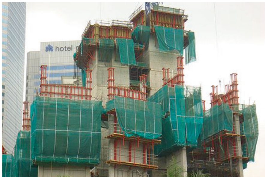
Fig. 1.27 The construction of Shear walls applying Rail Climbing System (RCS). http://www.perimalaysia.com/
