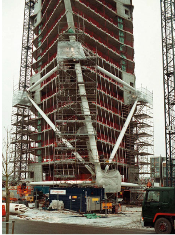
Fig. 10.4 Finishing panels to be pressed from the outside
