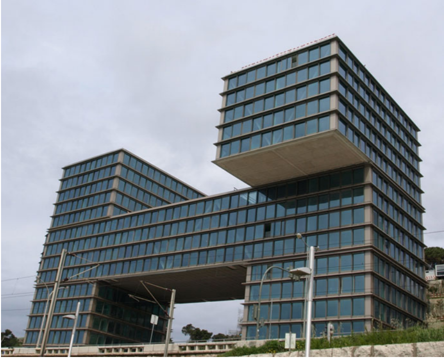
Fig. 5.1 A ‘glass tower’, recently built in Cascais, Portugal. Unfortunately, Glass Architecture is today fashionable, symbolizing economic status. It leads to excessive energy consumption (e.g., due to air conditioning), poor comfort levels, and damage to the environment. It is in flagrant contradiction with a truly sustainable design practice
