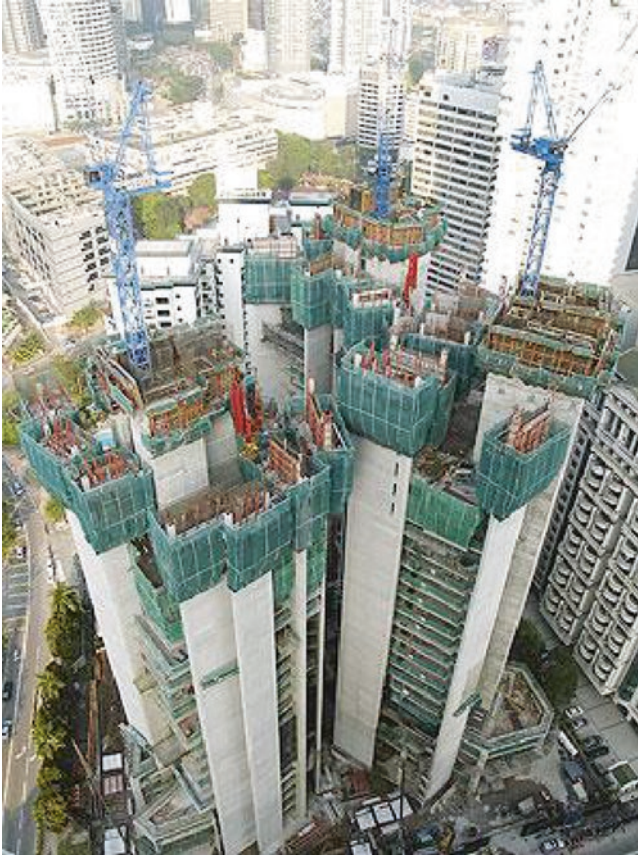
Fig. 1.26 The use of eco-friendly formwork, adapted VARIO system. http://www.perimalaysia.com/
