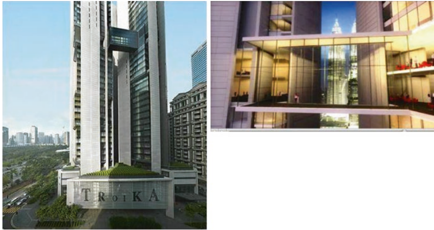
Fig. 1.16 The double-volume glass-encased bridges, an unique feature of TROIKA, with some 25,000 square feet of double-volume space spanning the three towers and connected by two sky bridges (Courtesy Aaron Pocock)
