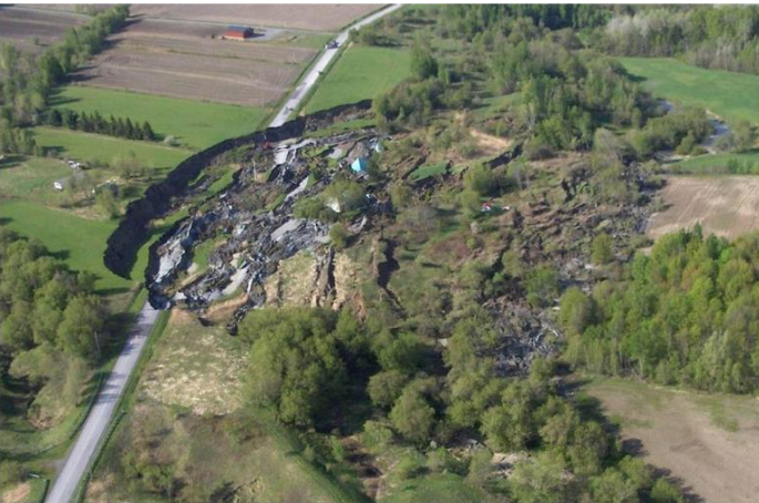
Fig. 17 a A lateral spreading failure following rotational sliding in extra-sensitive clay, St. Jude, Quebec, Canada. Photo Ministère des Transports du Québec
