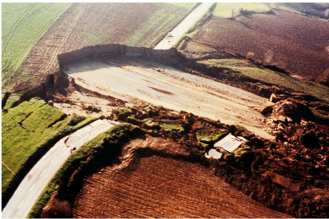
Fig. 11 A translational slide in tectonized Tertiary clay shale, Murazzano, Langhe district, northern Italy (Courtesy of Servizio Geologico della Regione Piemonte and C. Scavia, Turin Polytechnic)
