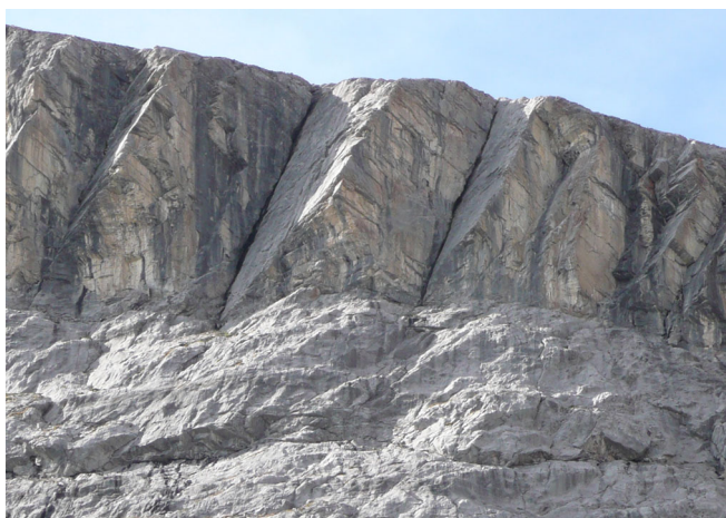
Fig. 8 Scars of wedge failures in limestone, Canmore, Alberta, Canada. The cliff is approximately 50 m high (Photo by O. Hungur)
