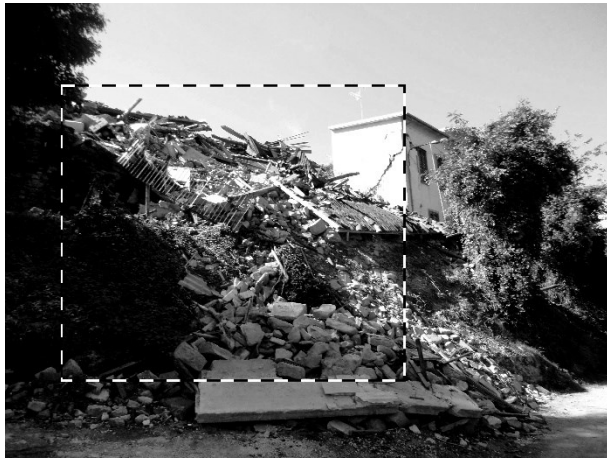
Figure 11: complete collapse of masonry wall (left) and (right) diagonal cracking due to shear failure (Amatrice).
