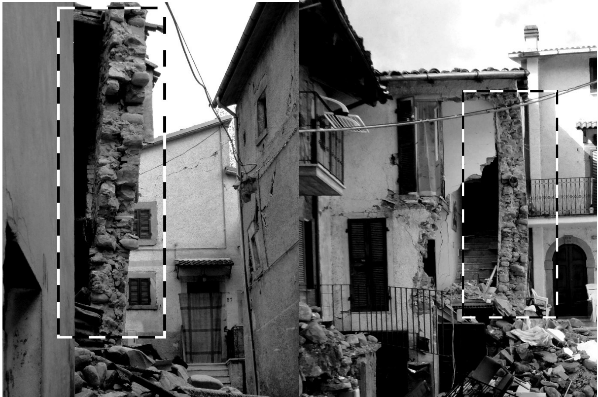
Figure 9: double wythe masonry wall (Accumoli).
