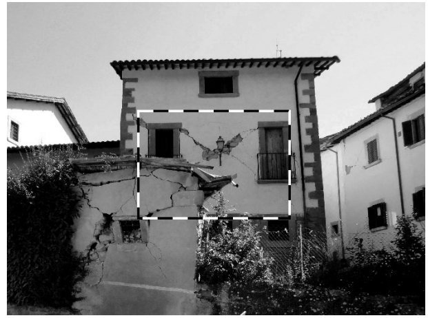
Figure 11: complete collapse of masonry wall (left) and (right) diagonal cracking due to shear failure (Amatrice).
