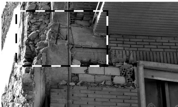
Figure 13: Beam-to-column joint failure due to lack of stirrups (left – Amatrice and right – Arquata del Tronto) (modified from ReLUIS, 2016).
