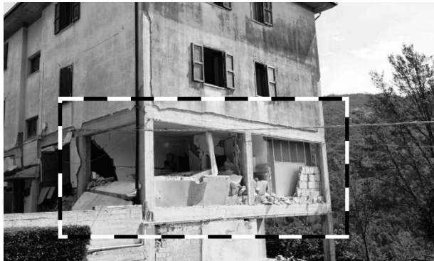
Figure 12: ejection of the infills (Arquata del Tronto - left) and soft storey mechanism (Amatrice - right) (modified from ReLUIS, 2016).
