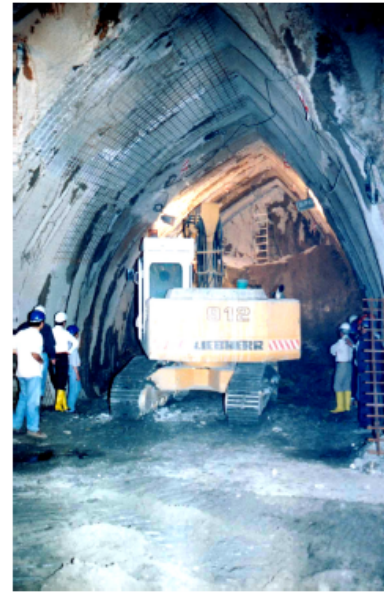
Figure 25: Twin side drift and central pillar excavation method. Temporary support consists of double wire mesh reinforced 250 - 300 mm thick shotcrete shells with embedded lattice girders or HEB 160 steel sets at 0.75 - 1 m spacing.
