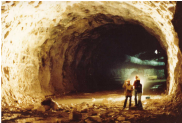
Figure 21: Top heading of the 12 m span, 18 m high tailrace tunnel for the Rio Grande Pumped Storage Project.
