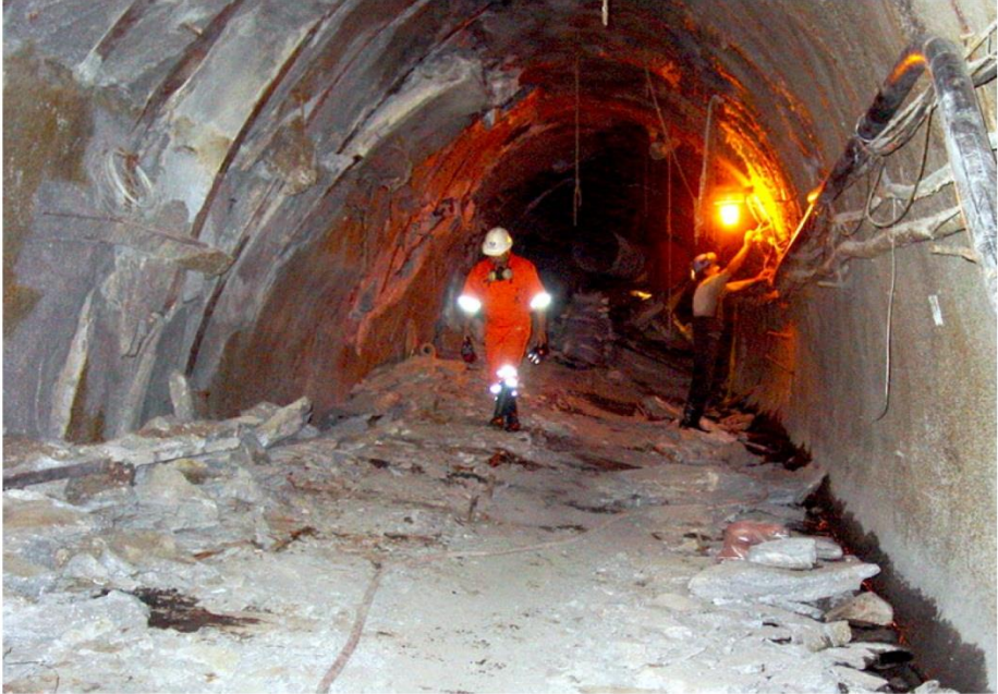
Figure 8: Failure of the lining in a horseshoe shaped tunnel in a highly stressed poor quality rock mass. This failure initiated at the corners where the invert meets the sidewalls.
