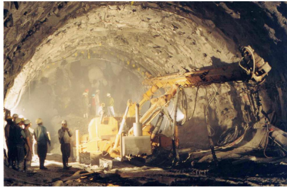
Figure 21: Installation of 12 m long 75 mm diameter pipe forepoles in an 11 m span tunnel top heading in a fault zone.
