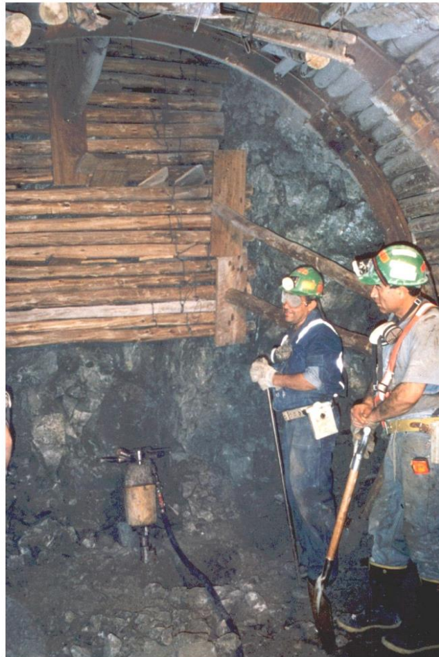
Figure 15: Installation of sliding joint top hat section steel sets immediately behind the face of a tunnel being advanced through very poor quality rock.
