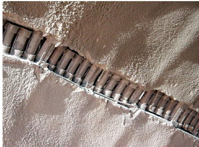
Figure 17: A row of stress controllers installed in a slot in the shotcrete lining in a tunnel
